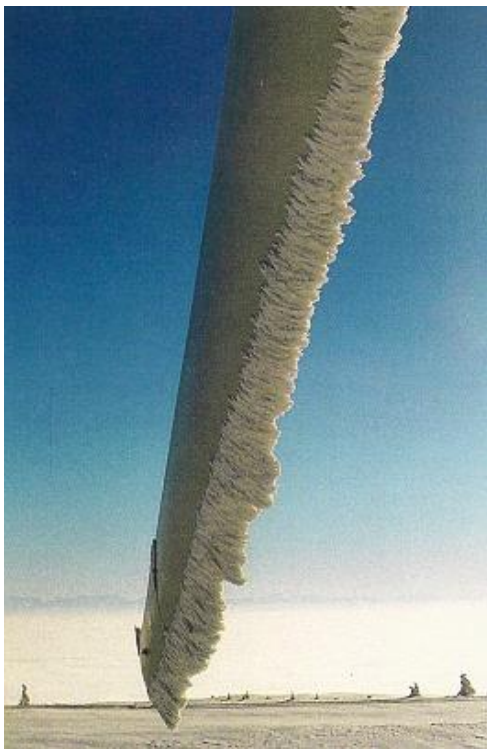
Figure 2-1 Icing on the leading edge of a wind turbine blade in Finland. The picture is shown with permission from the Finnish Meteorological Institute.
